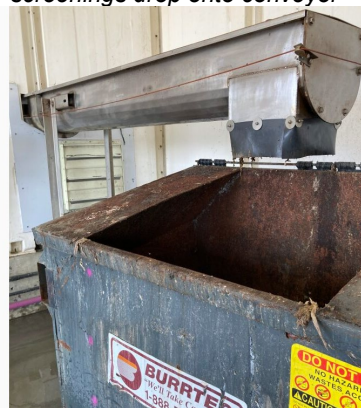
Compactor removed delivering direct from auger
