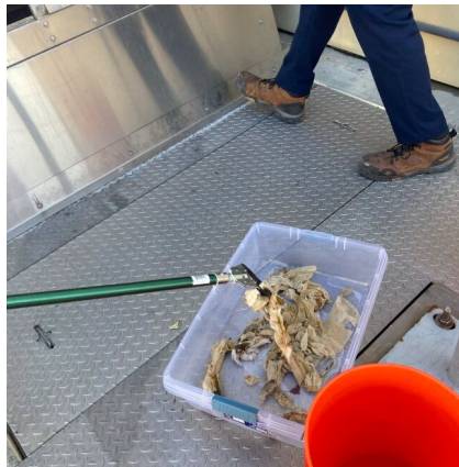
Placing screenings in tray
