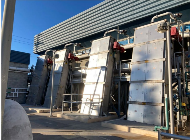
Four (4) screens with collection chute for screenings behind and gas extraction above.
