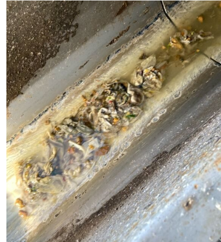
Slugs of screenings drop off a rake and flow down the chute before being captured in 5-gallon buckets with drainage holes drilled in them. Note the heavy intact organic load.
